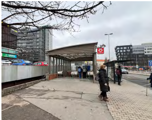
Figure 67 Canopy over the exit from the shopping arcade on the first underground level to the Poliklinika Budějovická stop, on Antala Staška Street. Author: ONplan, 2026
