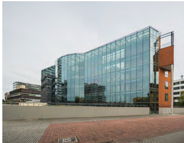
Figure 29 Poláčkova 1–976/2 office building. Author: ONplan
