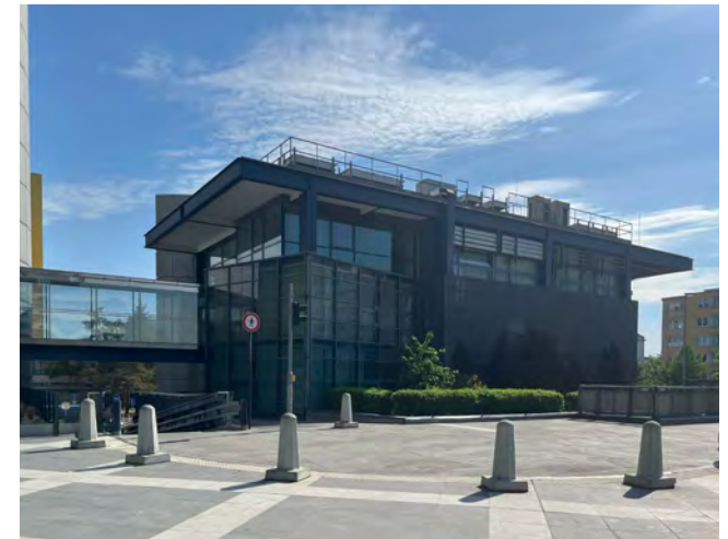
Figure 30 A small extension to the office building at Budějovická 1912/64b. Author: ONplan
