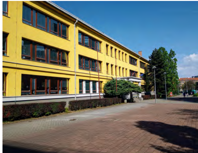
Figure 36 The main entrance to the primary school building on Poláčkova Street. Author: ONplan
