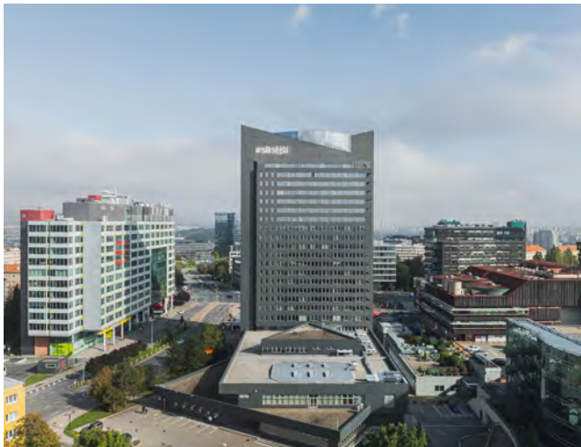
Figure 31 Office building at Olbrachtova 1929/62. Source: Penta Real Estate
