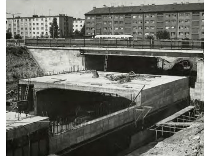
Figure 9 Construction of Metro Line C, showing the bridge over Olbrachtova Street, 1971. Source: 40 let DBK, 40let.dbkpraha.cz
