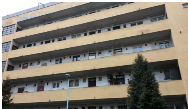
Figure 37 A balcony-corridor building from the 1930s in the Zelená Liška housing estate. Source: Praha Neznámá, www.prahaneznama.cz/praha-4/krc/zelena-liška/
