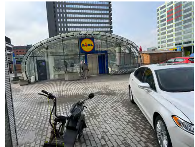
Figure 79 Photograph of the entrance to the Lidl building with a lift from the car park on the corner of Budějovická and Olbrachtova streets, providing a barrier-free connection between the shopping arcade on the first basement level and the street area at ground level. Author: ONplan, 2026
